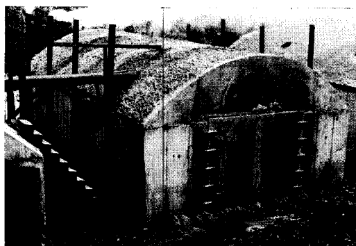
FIG. 1. A Missouri-type charcoal kiln. Burn is in progress. Majority of charcoal in the state is made in a kiln of this design.
