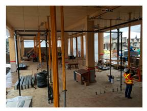
Figure 1. Type IV building under construction, using crosslaminated timber as part of the primary structure (image, Arup).
